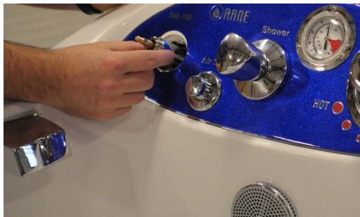
Step 11: Re-install part E (fig.1). Note: Do not over tighten.
