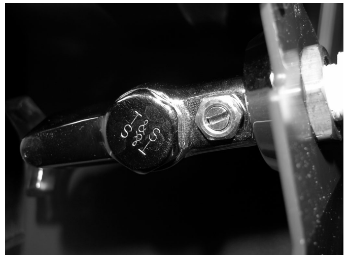
Water Flow Adjustment Screw
